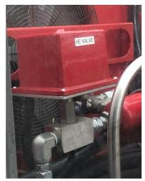
This valve actuator opens and closes a valve with the intake coming from the Booster Pump and the outtake going to the atmosphere on the side of the
