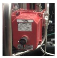
This valve actuator opens and closes a valve with the intake coming from the Pump and the outtake going to the intake of the Turbine Exhaust Heat Exchanger and to the atmosphere near the diesel tank. The button will control the valve if the system has power. It does not matter if the Valve Control is in Automatic or Manual.
