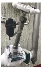
This valve is used to manual vent Nitrogen to the atmosphere from the heat exchangers on the N2 Tank.
