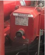
This valve actuator opens a valve with the intake coming from the Pump and the outtake going to the intake of the Turbine Exhaust Heat Exchanger and the intake of the Turbine Intake Heat Exchanger. The physical button will control the valve if the Valve Control Selector Switch is set to Manual mode. If the Valve Control Selector Switch is set to Auto mode, the PLC will control
