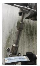
This valve allows Nitrogen to travel from the check valve from the heat exchangers on the side of the N2 Tank to another check valve toward the atmosphere dump.
